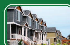
REAL ESTAT Real Estate Activities
